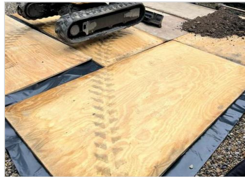
Plywood laying on gravel ground
